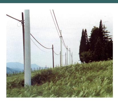
ICP GRP composite poles (a technical combination of glass and resin) are a high-tech innovative product, which can withstand high stress and all known atmospheric conditions. The poles are made of orthophthalic unsaturated polyester resins and reinforced by fiberglass rovings, mats or fabrics. The exterior is made of polyester resin treated for ultraviolet stability.
